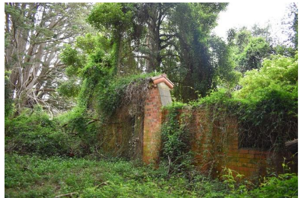
Figure 43. View of the brick fence and wrought iron gate.
