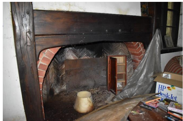
Figure 40. Detail view of the fireplace.
