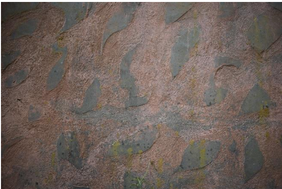
Figure 25. Detail view of the cement render.
