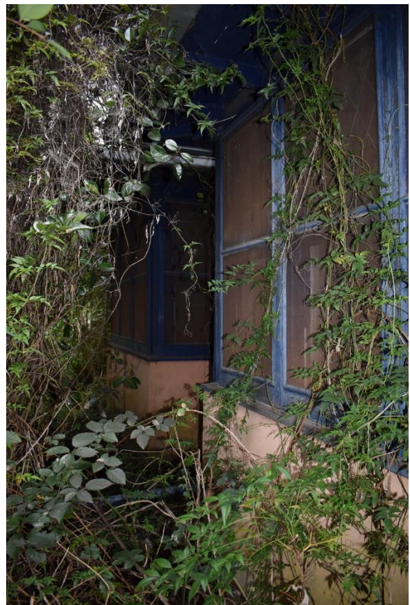
Figure 30. View of the projecting, expressed timber framed windows from the courtyard.
