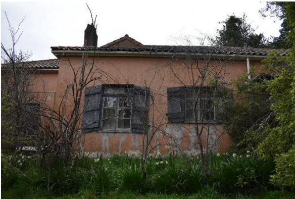
Figure 17. View of the western elevation of the house.
