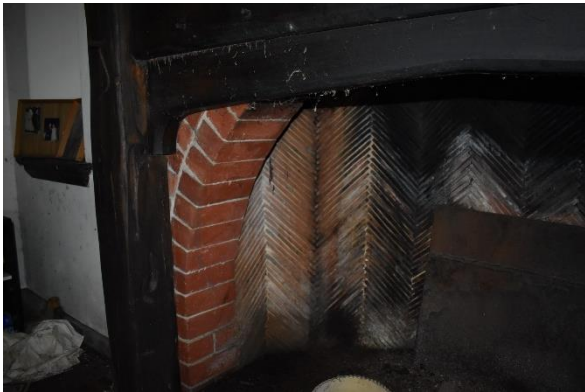
Figure 41. Detail view of the fireplace.
