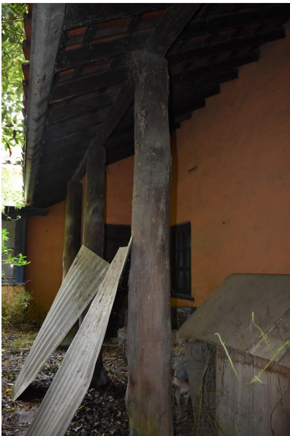
Figure 29. View of the southern verandah and bush poles.
