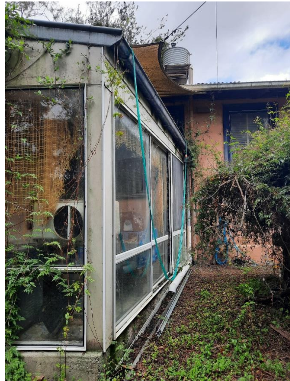
Figure 24. View of eastern side 1980s alteration. Source: Yarra Ranges Council.
