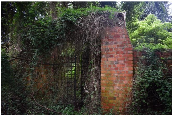
Figure 42. View of the brick fence and wrought iron gate.
