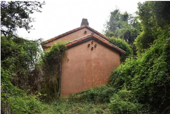
Figure 15. View of the western section of the house from the south.
