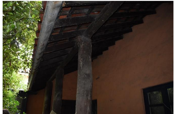
Figure 28. View of the southern verandah skillion roof and bush poles.
