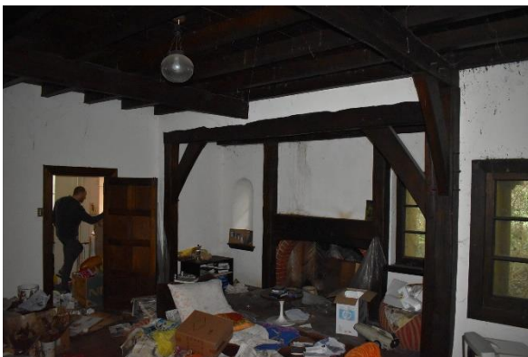
Figure 37. Interior view of the Dining Room including fireplace.
