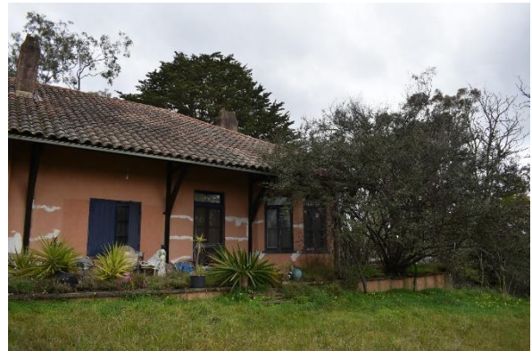
Figure 18. View of the northern elevation of the house.
