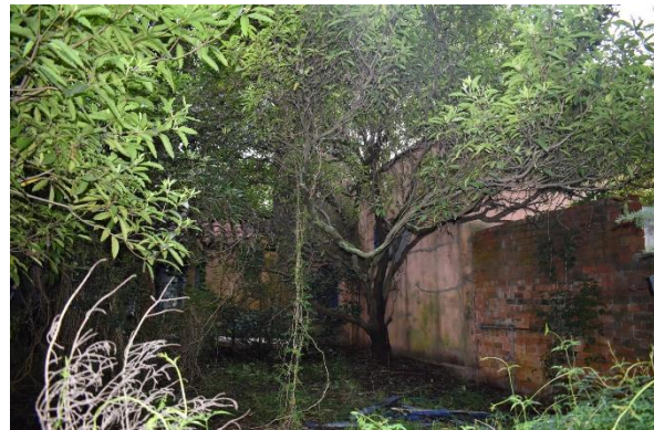
Figure 26. View of the courtyard and house from the south.
