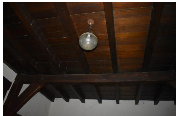
Figure 38. Detail view of the ceiling.
